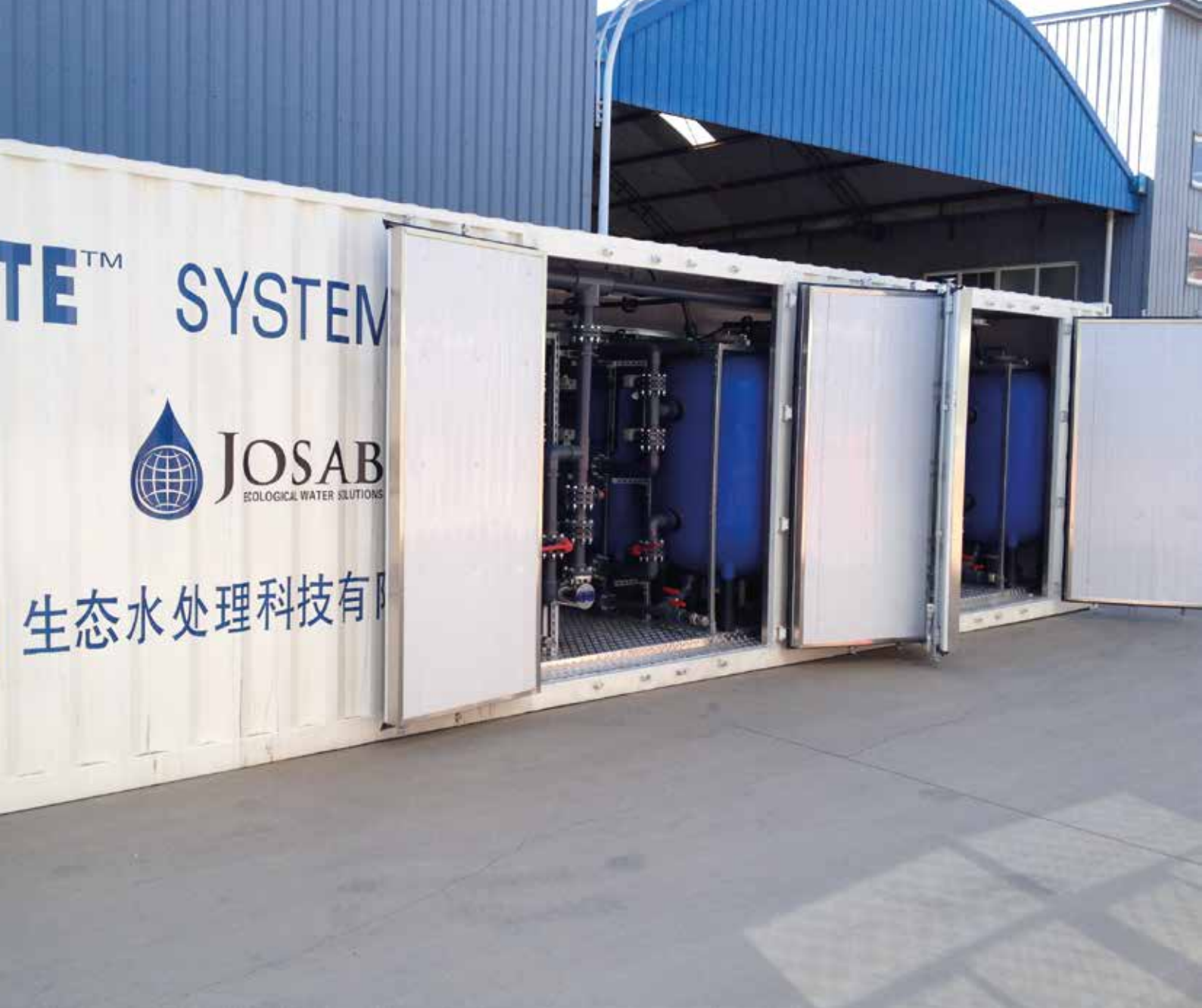
Entry doors to the 2 Side Opening modules mounted in a SC1800 for a Chinese customer
