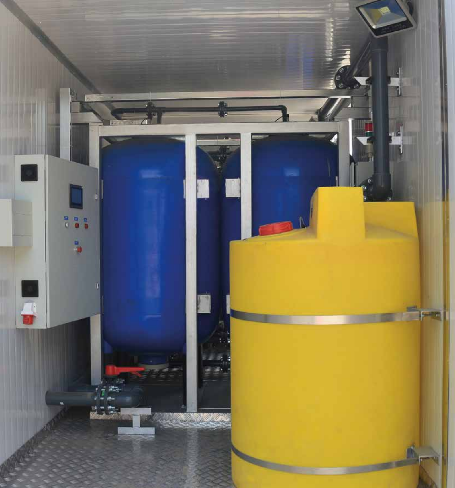
Monitor section of the SC900E (electric) with control cabinet and chlorine injection
