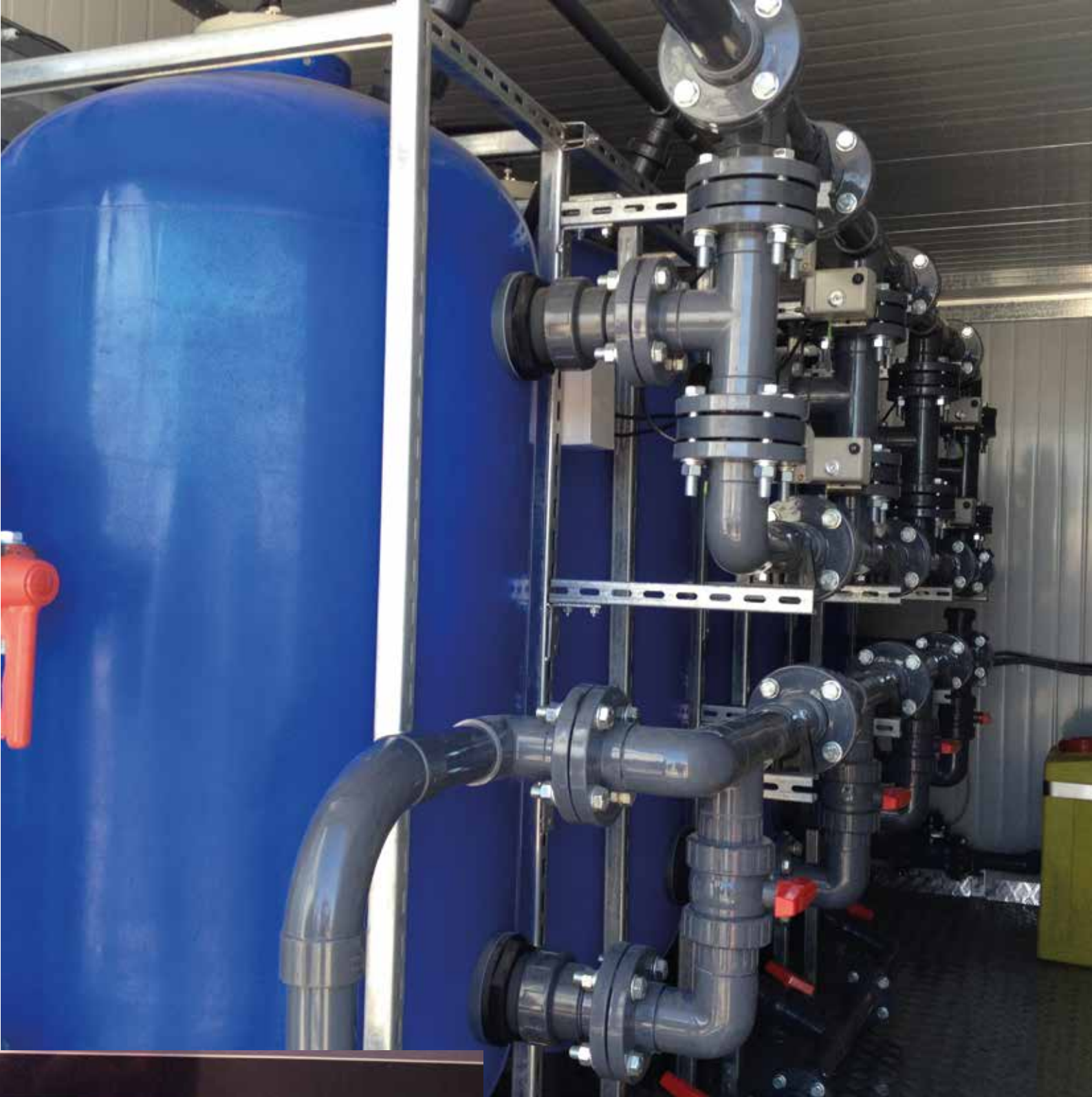
SC500E (electric) a full automatic controlled unit, with electrical valves and full-colour touchscreen control display.
